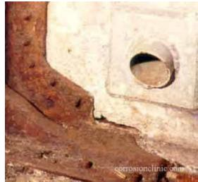
The most severe attack occurs at the joint between the two dissimilar metals. Further away from the bi-metallic joint, the degree of accelerated attack is reduced.
